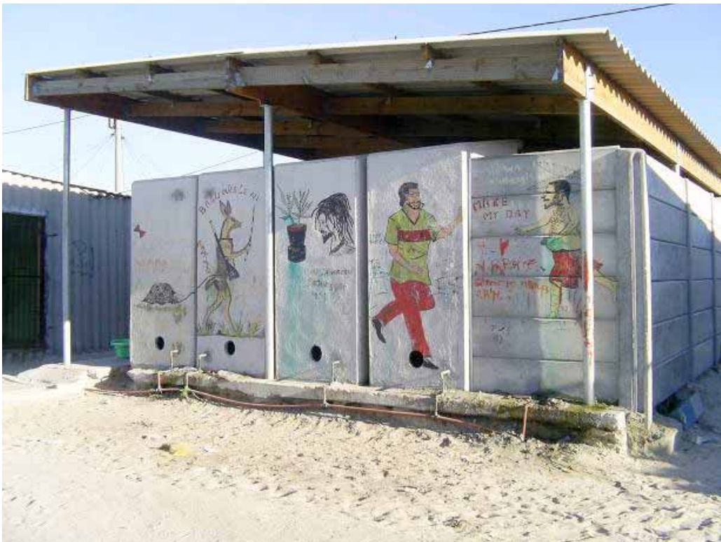
Figure 7: Communal ablution block in Tsunami
