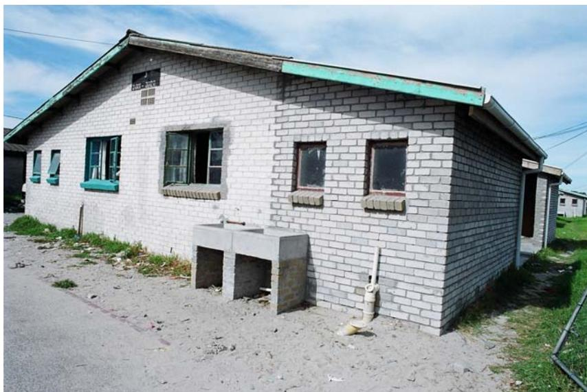
*Figure 4: Bokomo Hostel in Nyanga; the design and layout of the blocks made it possible for each block to be converted into four attached dwellings each on its own plot with road access.*
