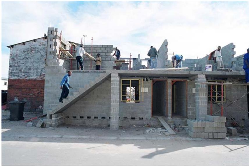
*Figure 11: Construction of an infill block in the hostels redevelopment programme in Langa*
