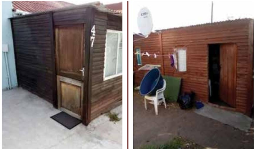
Figure 9: Typical backyard structures made of timber panels.
