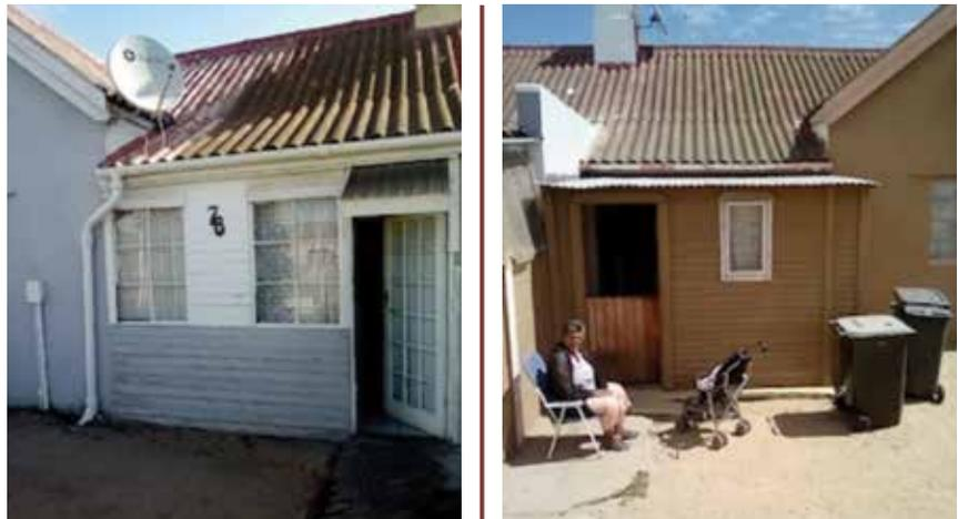
Figure 8: Typical main house structures. In both instances with porches filled in to expand the original building.
