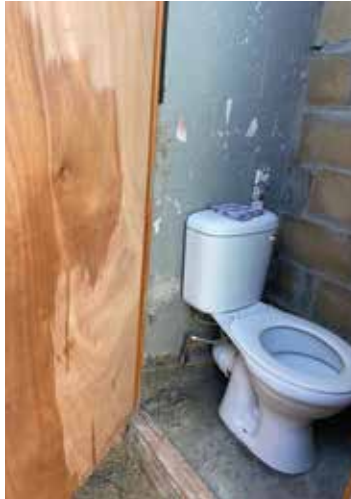
Pictured above: The new toilet installed outside.
