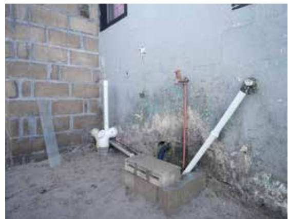
Pictured above: Installed communal tap and sanitation pipes.
