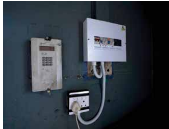
Pictured above: After the new installed box inside the main house.
