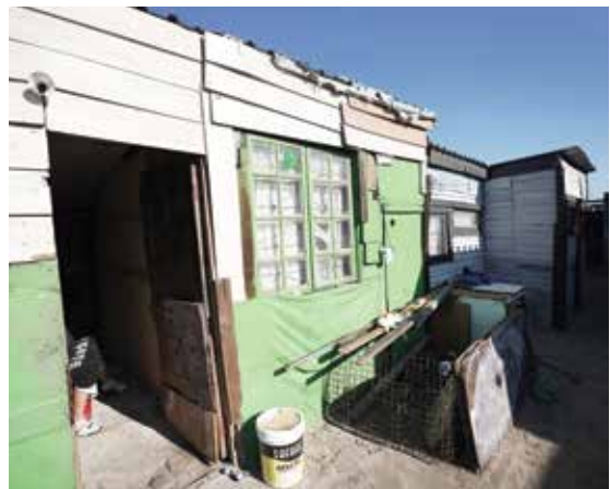
Pictured above: One of the five backyard structures in the yard.
