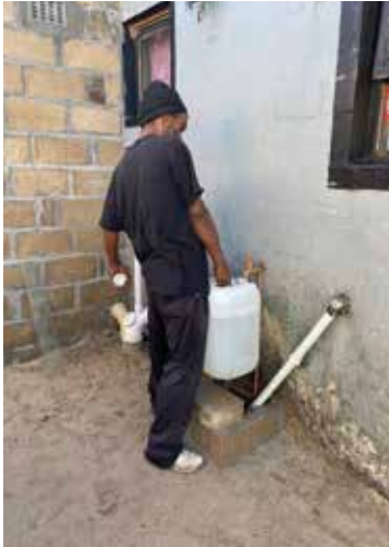
Pictured above: Tenant using water from the new installed communal tap.
