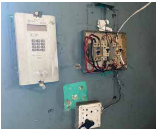
Pictured above: The before condition of the main house electric box.
