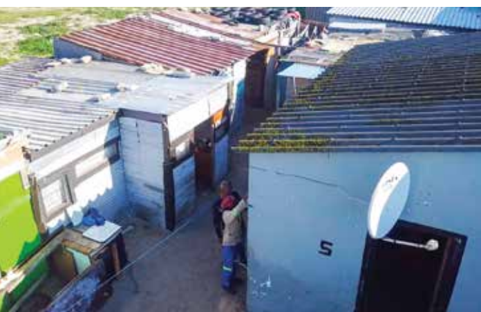
Pictured above: Certified electricians installing services.
