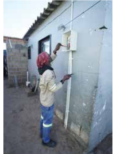
Pictured above: Certified electrician installing the electric box.
