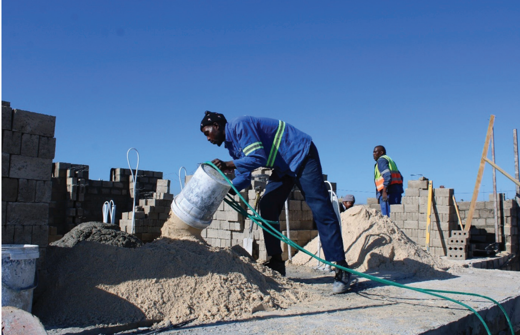
Pictured above: Emerging contractors on site during the construction phase of a small-scale rental housing development.
