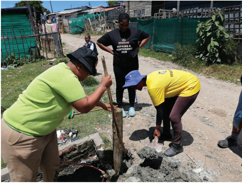
Pictured left: Task team members installing a standpipe.
