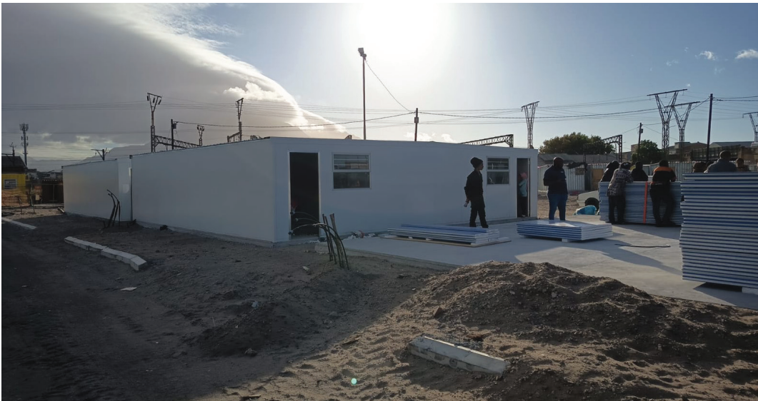
Pictured above: The construction of the first permanent structures in Phase 2 at Ghost Town (Maitland Intersite).
